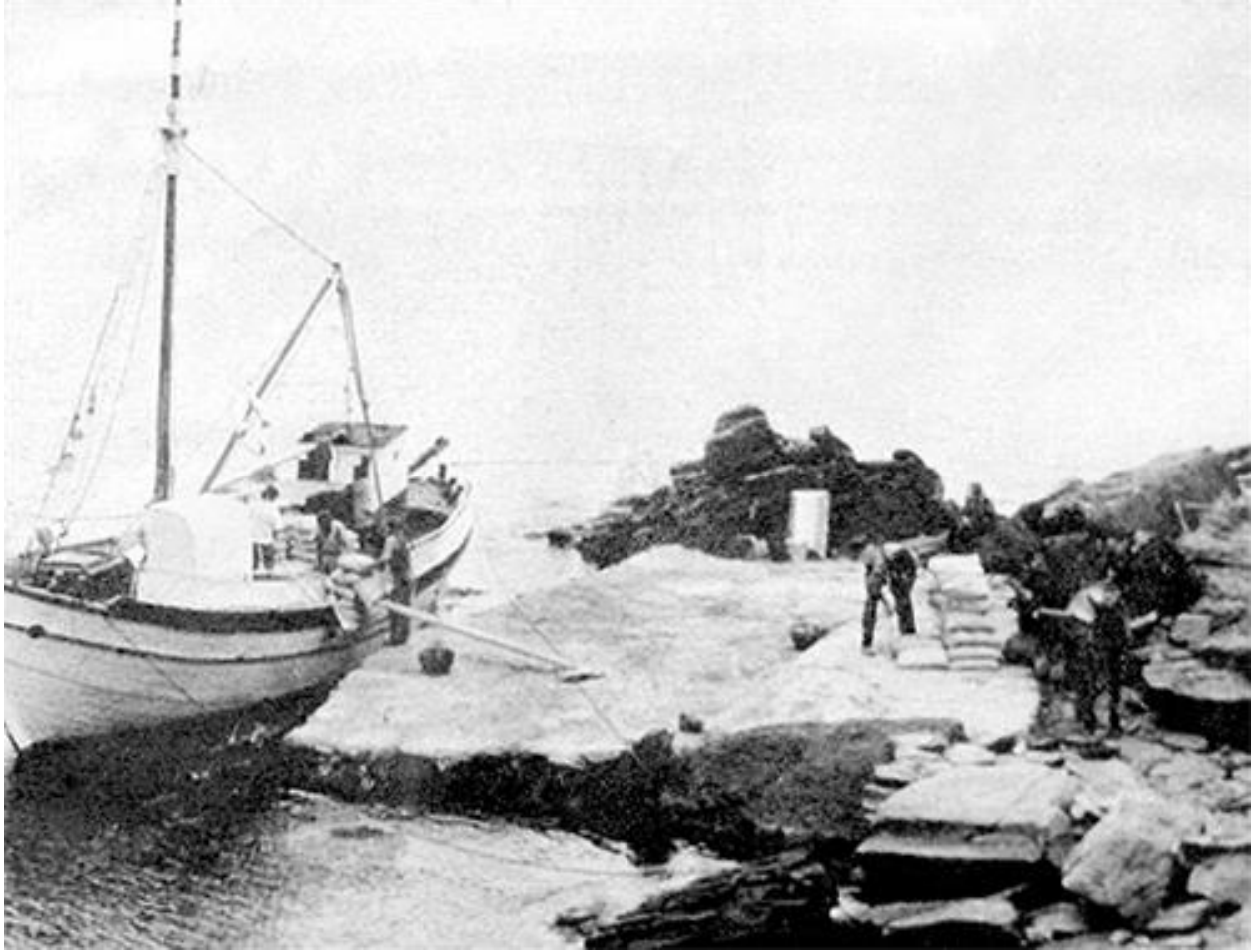
7.5 The dock that lasted twenty-four hours at Klima
